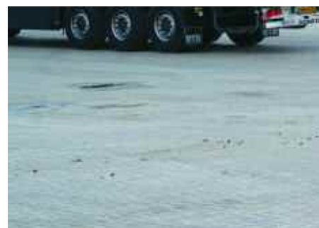
Block paving is chosen over concrete for outside yard space at both Renners and Rehhütte – it costs the same to lay, but it's more flexible.
