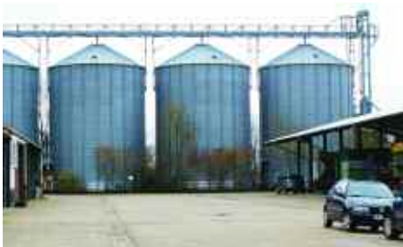
All of the combinable crops are stored at Rehhütte in 650t silos.
