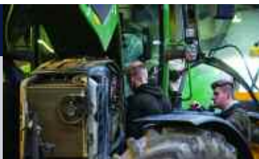
Some control boxes are susceptible to low voltage, so it can be best to wire straight off the tractor battery.
