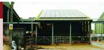
A roof-mounted solar array and harvested rainwater have slashed energy bills.
