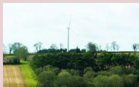
Electricity is fed to the community from the estate's 500kW wind turbine that sits high on a hill.
