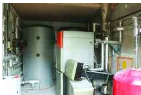
Woodland on the farm is sensitively managed with thinnings processed and used as fuel for biomass boilers, displacing around 160kWh/yr from fossil fuels.
