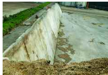
The 23° Ark sloping walls of the clamp also allow for safe piling of material above the height of the panels and enable machinery to work right up to the edge.
