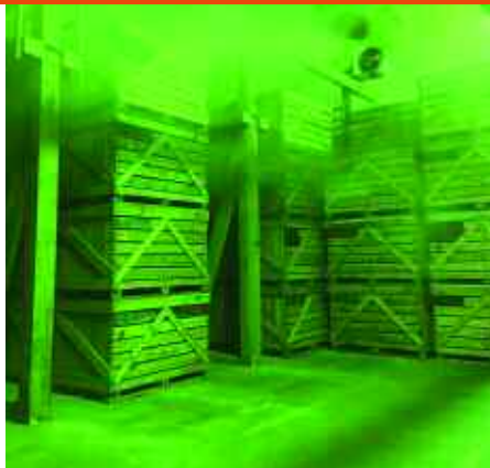
Fogging application rising to the top in store.
